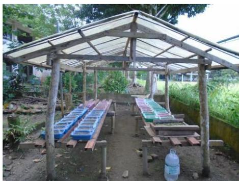
**Figure 1.** The coco lumber and bamboo were used plastic transparent 'UV' film in the roofing.
